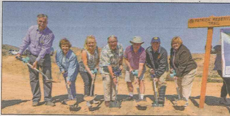
Breaking ground for the Trekking Catalina trail expansion project. Pictured above from left to right are: Tony Budrovich (Conservancy President and CEO), Ann Muscat, PhD, (Immediate Past Conservancy President), Alison Wrigley Rusack (Conservancy Benefactor Member), Supervisor Don Knabe (County of Los Angeles, Fourth District), John Cotton (Conservancy Past Board Chair and IMAGINE CATALINA Co-Chair), Dan Knapp (Executive Director and CEO, Conservation Corps of Long Beach) and Jane Beesley (District Administrator, Los Angeles County Parks and Recreation and Open Space District). Photo by Robb Rosenfeld
